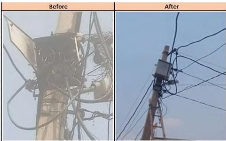
Conversion of Old Bare Conductor to OH Armoured Cable with Pole Top
